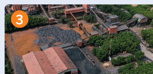
Ananthapur Unit-II, Andhra Pradesh
